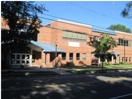
North East Façade and Main Entrance
