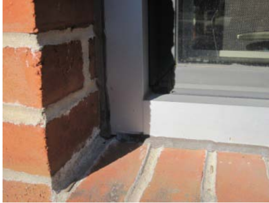
Caulking around perimeter of window framing in good condition
