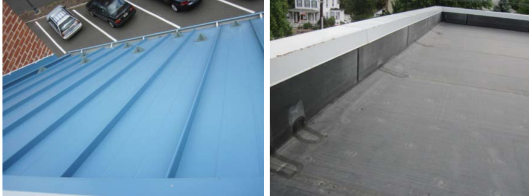
Standing seam metal roof and single ply EPDM roof membrane
