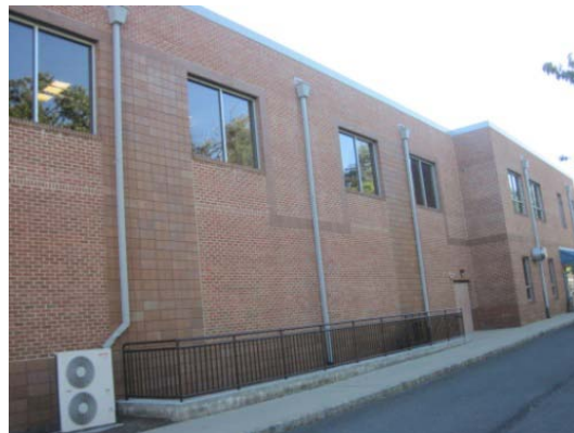
South West Façade
