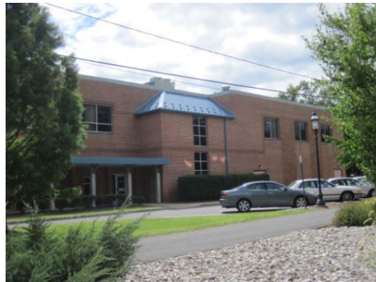
North West Façade
