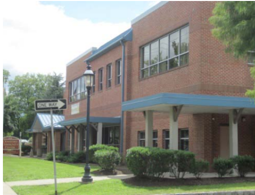
North East Façade – typical exterior walls
